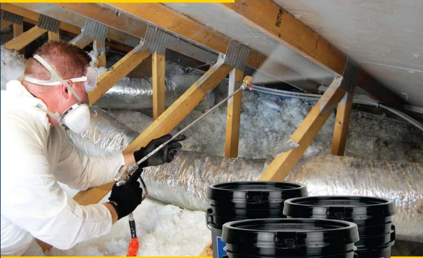
Henry LiquidFoil Attic Barrier is a radiant heat control coating that keeps heat out of a building during the summer and in during the winter. By keeping approximately 84% of radiant heat from entering or escaping a building, LiquidFoil Attic Barrier can cut energy consumption and costs significantly. It's as easy to apply as paint and dries quickly to a shiny, metallic finish.
