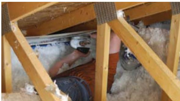
Stapled in place sheet applied or foil radiant barriers can be difficult and time-consuming to install in existing home attics.
