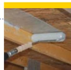
Can be applied using a roller applicator
