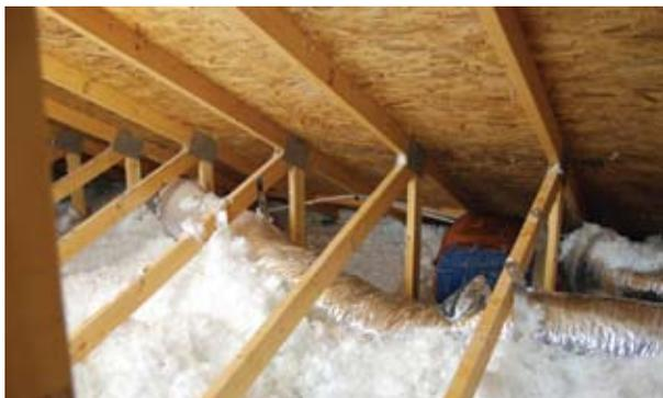
Installing insulation can involve cramped and uncomfortable working conditions as well as hazardous fiberglass fibers.
